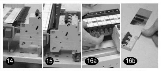
Note: Install MCB with white DIN rail clip facing busbar (i.e.) MCB switches 'off' towards busbar.
